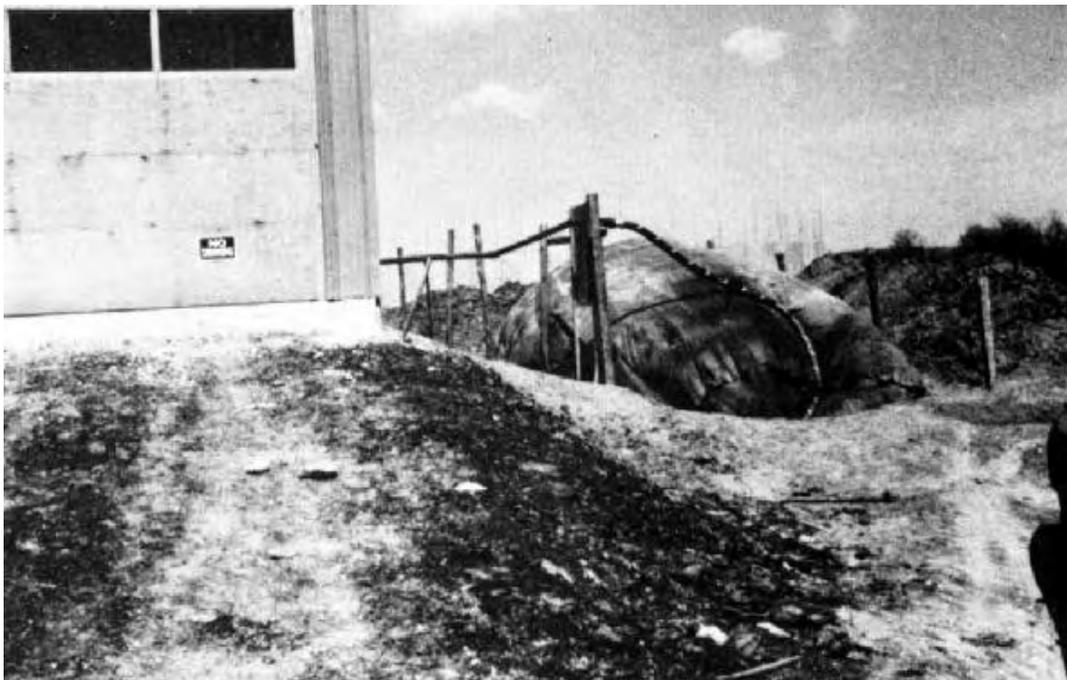
**Figure 8. Flexible storage bag for methane gas**
