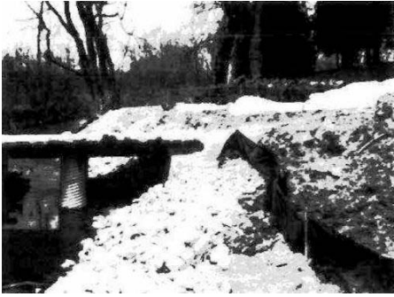
Fig. 12. Temporary seeding during construction shut down - Before.
