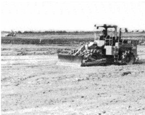
Fig 7. Grading on construction site.
