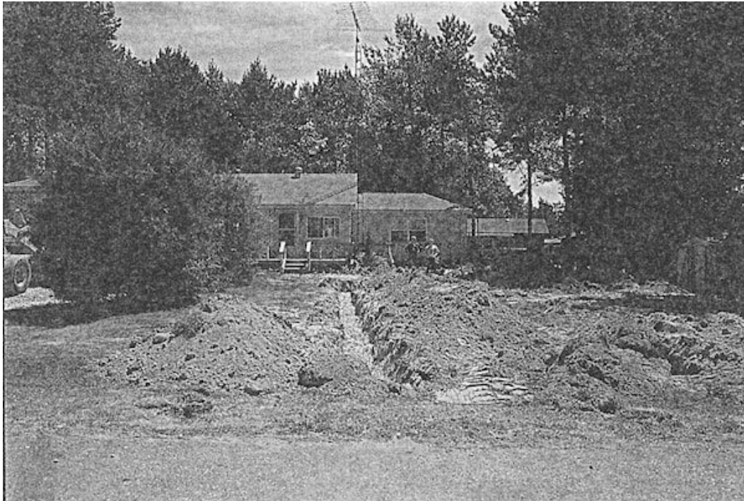
Figure 6: Weeping bed installation near Innerkip
