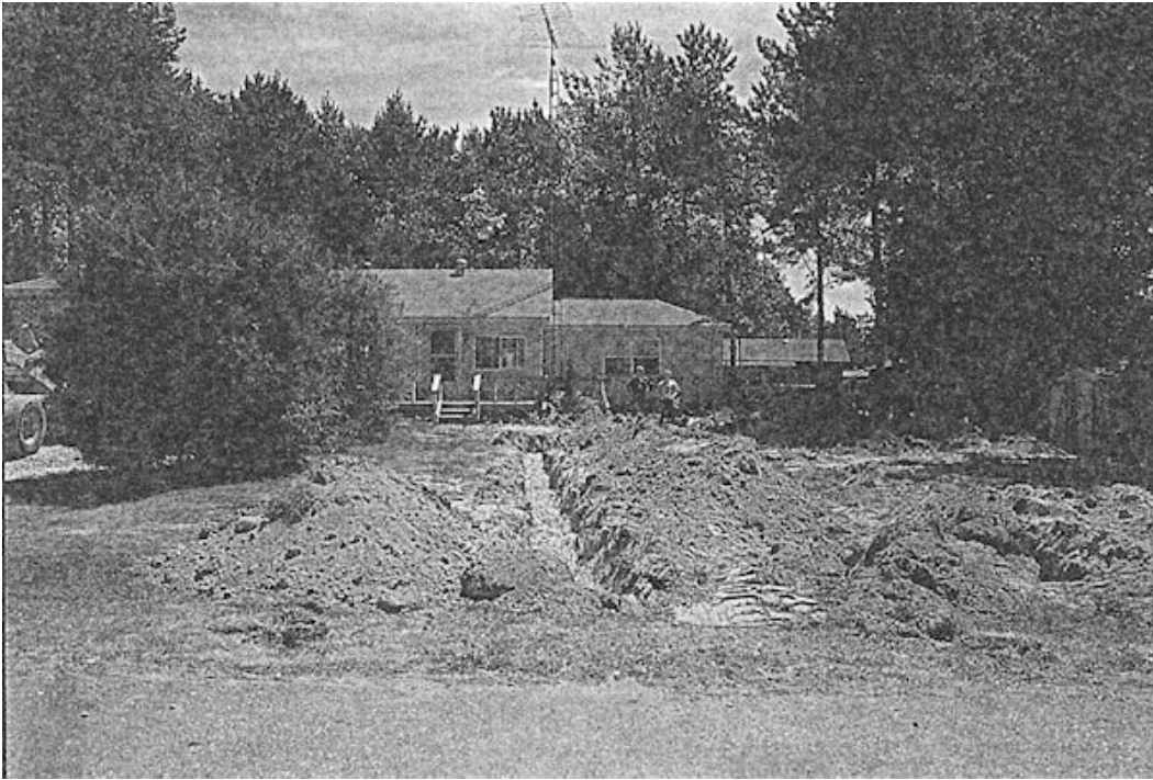
Figure 6: Weeping bed installation near Innerkip
