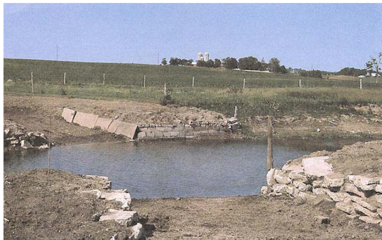
A controlled cattle access which was constructed from materials found on most farms.
