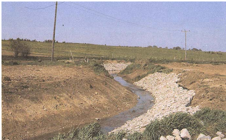
An open drain with properly sloped and protected banks.
