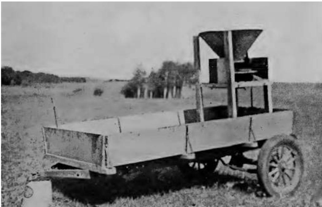
**FIG. 7.** Autotrailer bait spreader.
