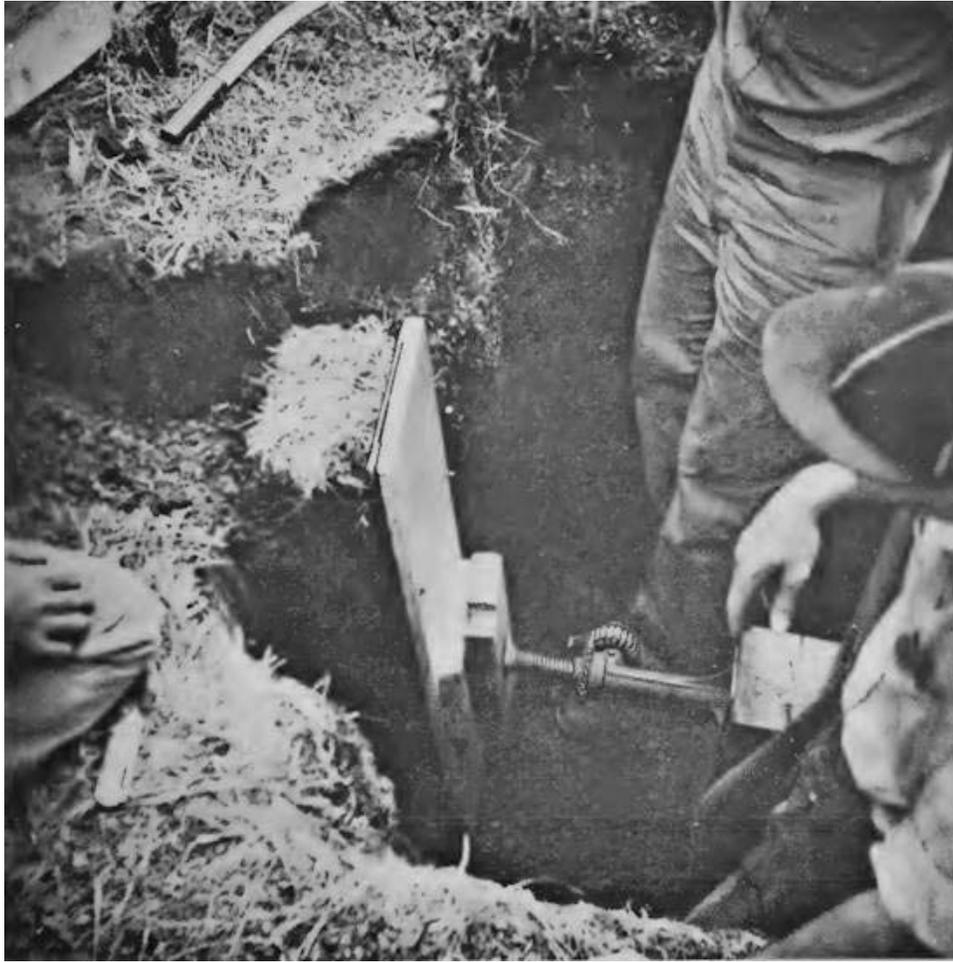
**Fig. 4.** When the backing board is in place, the soil is dug away from the sides and back of the column.
