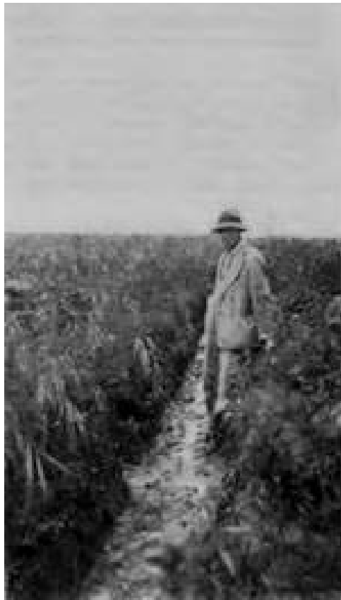
View of lateral ditch. Peat land reclamation project. Caledonia Springs, Ont.
