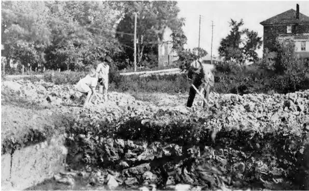
View of peat deposit showing underlying bed of marl, Ottawa. Canada.
