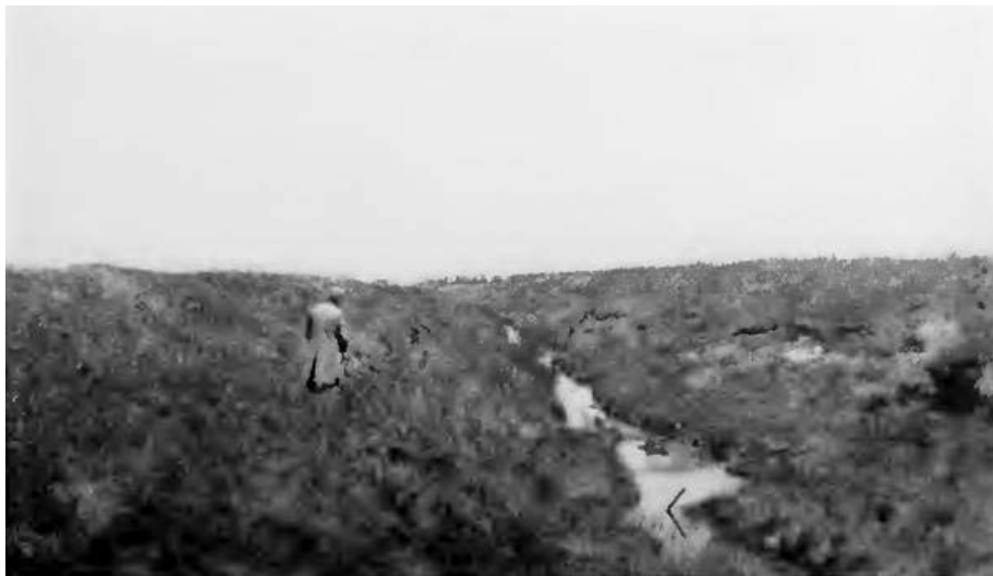
View of main drainage ditch. Peat land reclamation project, Caledonia Springs, Ont.
