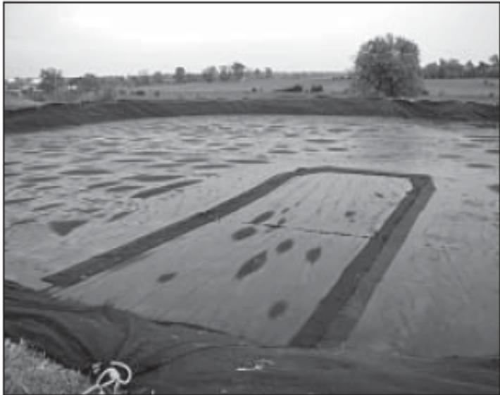
**Figure 2** Opening for the access of agitation and pumping equipment in a geotextile-covered manure storage (Bicudo et al., 2003)
