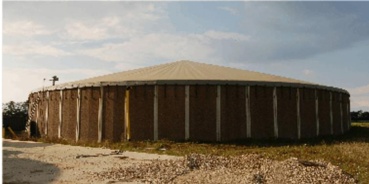
**Figure 12** Plastic cover supported by central pillar and series of guy ropes
