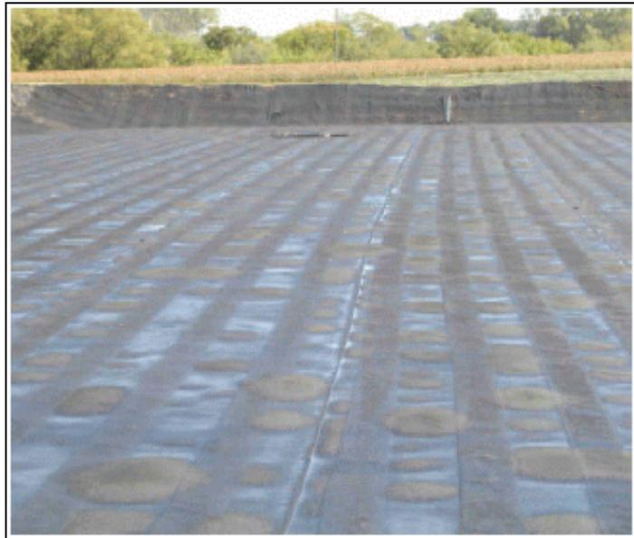
**Figure 3** Geotextile floating permeable cover with closed-cell floatation (Nicolai et al., 2002)
