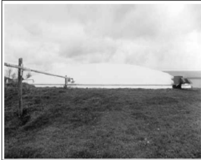
**Figure 5** An Inflatable cover on the top of a 23 m diameter concrete manure storage tank (Zhang and Gaakeer, 1998)
