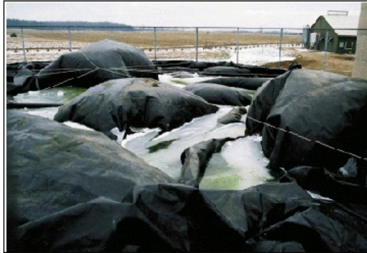
**Figure 11** The negative air pressure cover during manure agitation by forced air in early winter (Barry, 2006)
