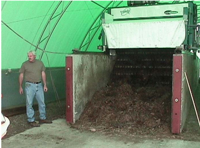
Figure 7. Turner at end of channel - partly composted straw + pig manure.
