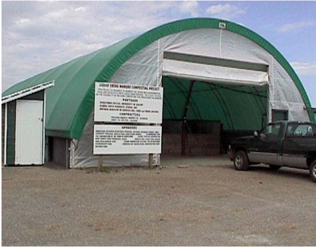
Figure 1. Building housing the compost channels and mechanical turner.
